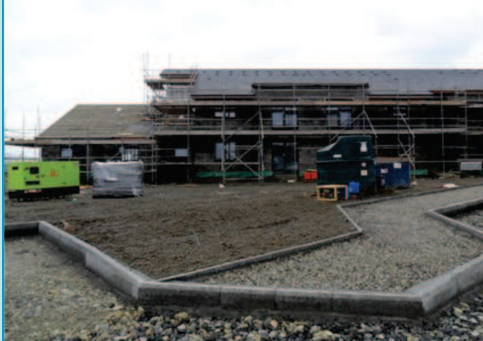
Mull Progressive Care Centre under construction
